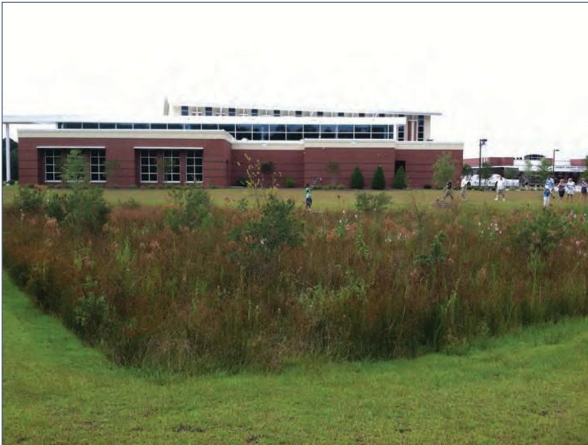
Figure 4.52 Stormwater Wetland at Carolina Forest Recreation Center, Myrtle Beach (photo: Kathryn Ellis).
