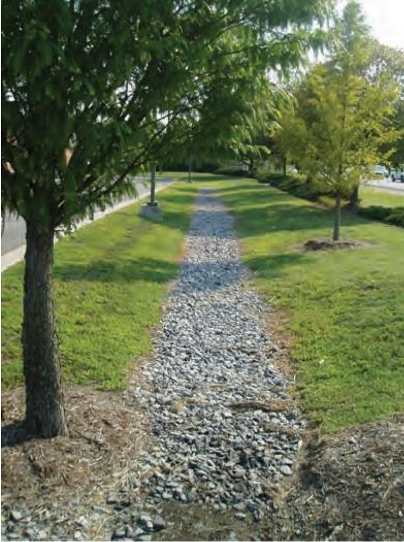
Figure 4.16. Infiltration practice in median strip.
